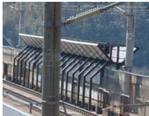
Image 3: Y-shaped noise reduction fence
